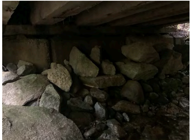
Right Bank Abutment when facing downstream
