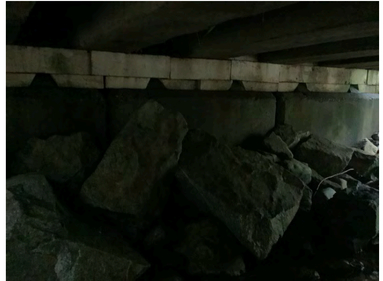
Left Bank Abutment when facing downstream
